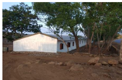
Ongoing renovation at the Ashramshala support Project
